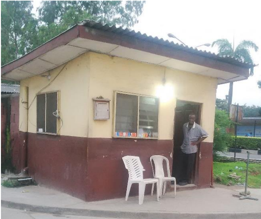
Plate 1: A Typical Security Post in the University of Lagos Source: Fieldwork, 2016
